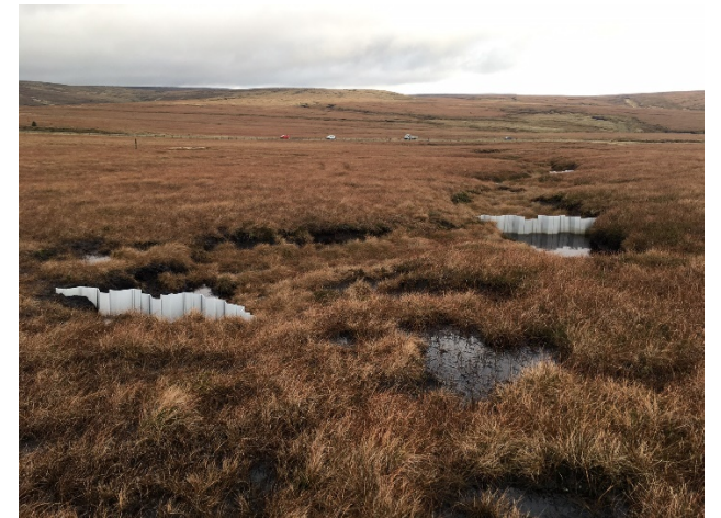
Gully blocking south of A57
